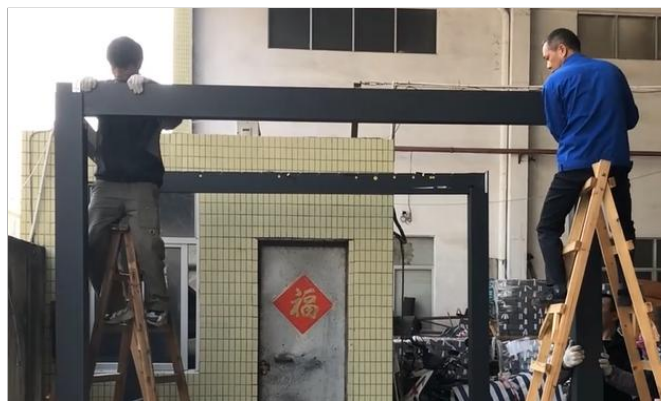
11. Pay attention to the fact that the beam is the same length as the motor beam, and the one with a row of mounting holes is the opposite beam, and the rest is the ordinary beam
