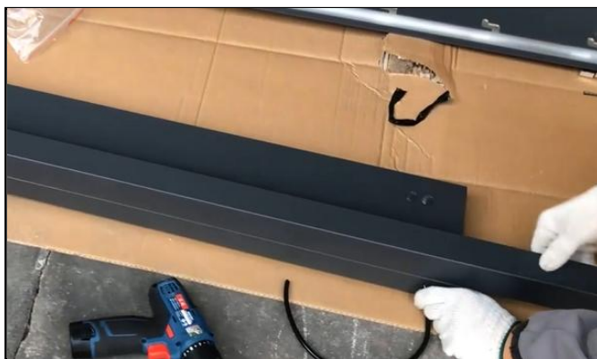
10. Continue to install the remaining beams and built-in sinks in the same way
