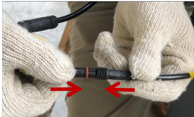
8. Connect the labels of the light belt and motor line on the beam to the lines with the same labels on the column. After the connection is completed in the direction of the arrow, put the lines back into the column
