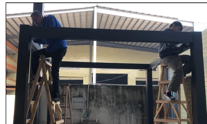
12. all beams after installation should remember to lock the connecting block, if there is an optional windproof shutter, should be installed after the completion of the beam, start to install windproof shutter.
