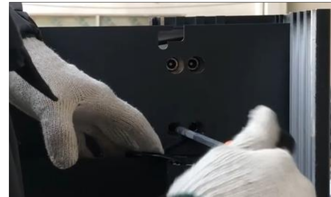
9. Lock the beam coupling block with the hex wrench.
