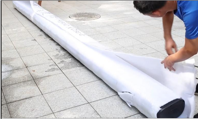
1. Open the package carefully to avoid scratching the awning
