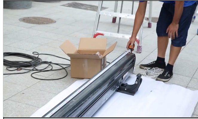
2. Measure the total length of the awning
