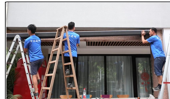
12, hang the awning (careful product weight, it is recommended to operate more than one)
