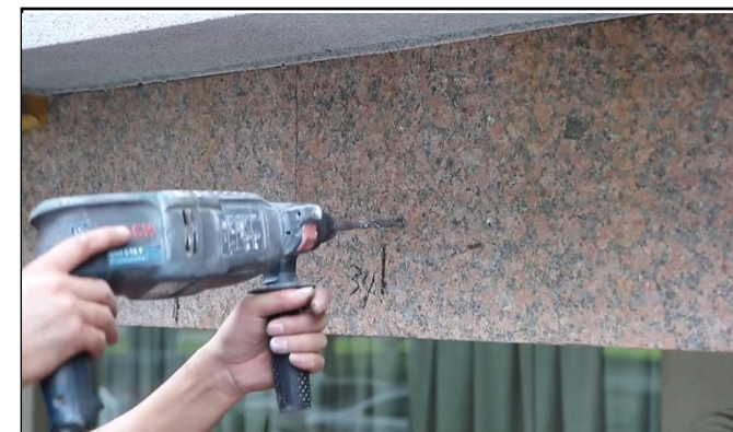
9. Drill out all screw holes with a hammer drill
