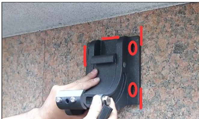
8. Measure with a level and mark the position of each wall code and the position of expansion screws.
